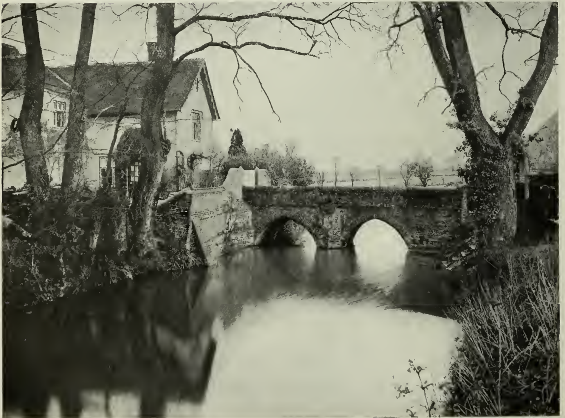
STEEPLE BUMPSTEAD: LATCHLEY'S MANOR HOUSE.
